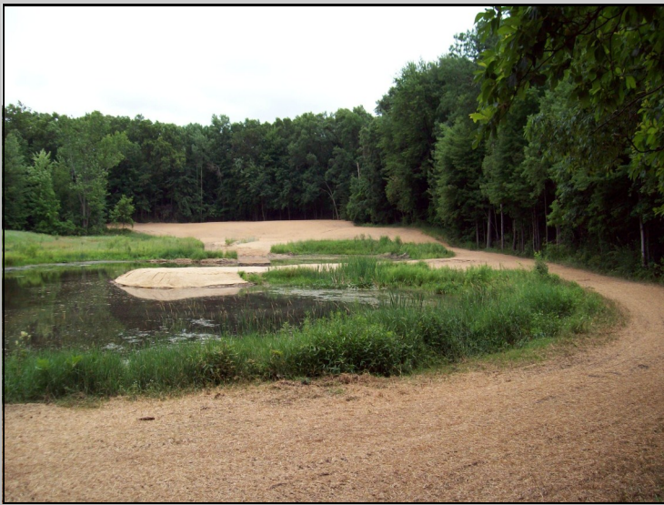
Wheeler Sediment Basin after cleanout
