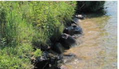
This encapsulated soil lift and the established native shoreline vegetation stabilize the shoreline – even with moderate to high wave and ice action. Encapsulated soil lifts also slow runoff from upland areas, improve fish and wildlife habitat, improve water quality, and deter geese from damaging property. Photo courtesy of Michigan Natural Shoreline Partnership.
