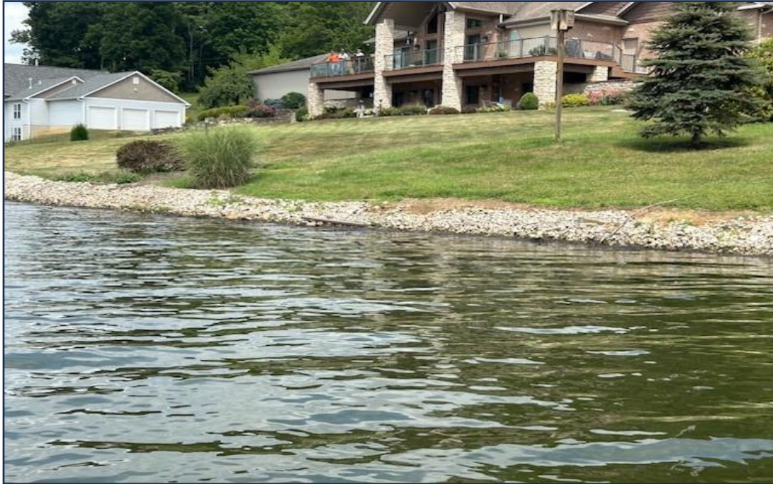
Figure 13. An example of a lake shoreline home with riprap to reduce erosion (2024).
